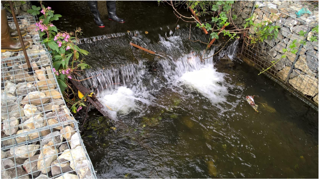
Figure 3 – Section 2: Concrete weir
